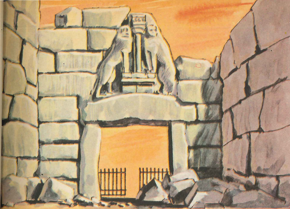
The Gate of the Lions at the entrance of Mycenae, a city in southern Greece, dates from 1200 B.C. and is based on the beam and lintel principle.
